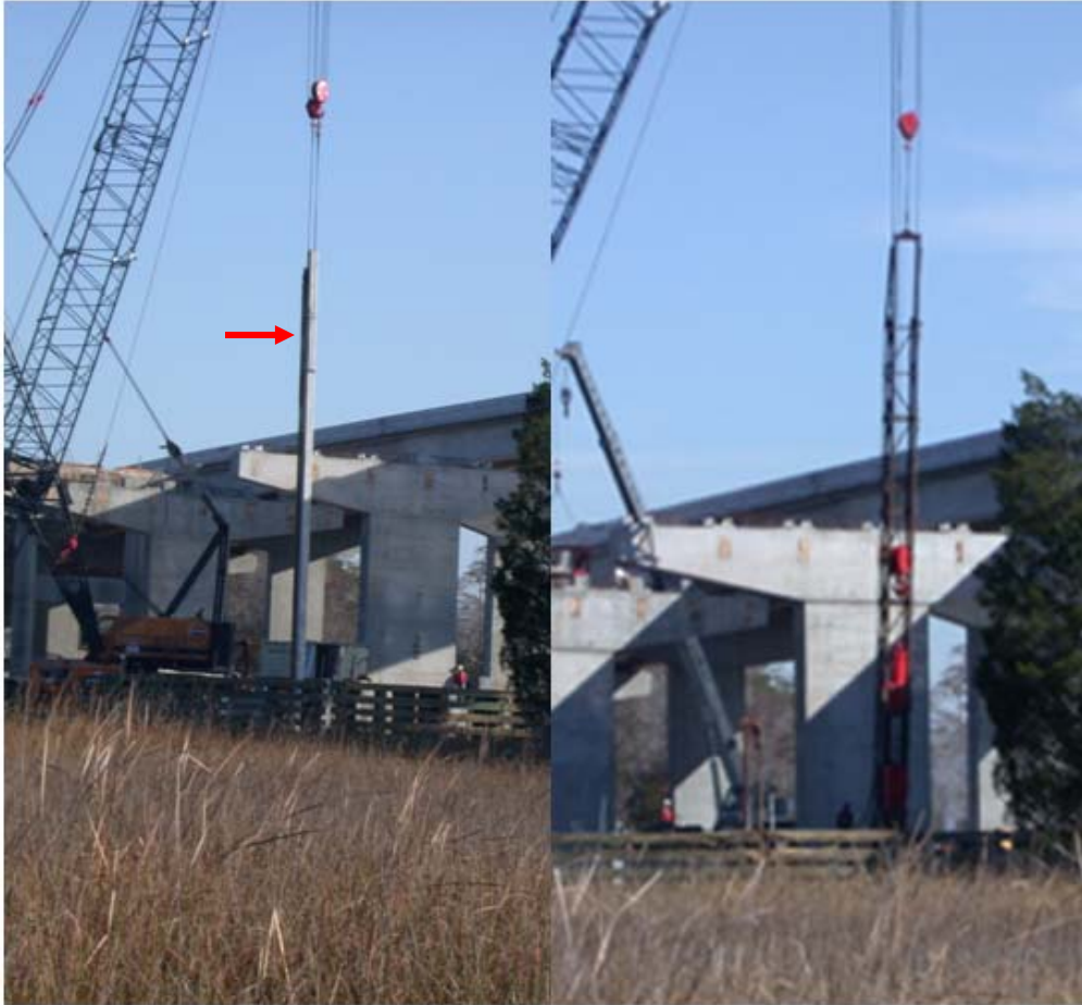
Figure 1.3.6-2. Construction activities at new US Highway 90 bridge over Escambia River. At the left, red arrow indicates pipe attached to piling that channels water to the water jet. To the right a pile driver being used to drive pilings is suspended from a crane. (Photos C.J. Mohrherr, Jan. 2004).
