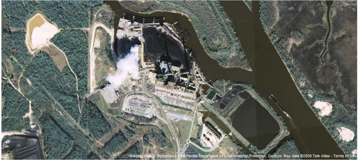
Figure 1.4.6-1a. Aerial view of Crist Steam Plant on Governor's Bayou and Escambia River.
