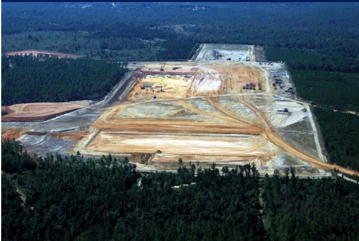
Figure 1.4.9-1b. Site progress at location of new ECUA treatment plant as of October 2008 (ECUA, 2008)
